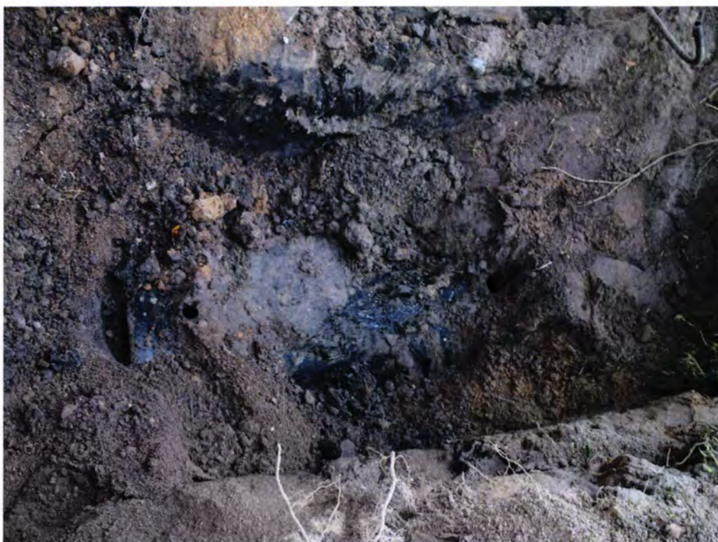
Picture 2: UST 774Althea removal in progress.
